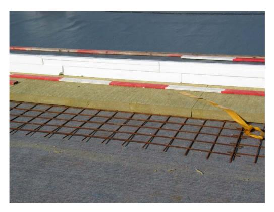
Fig. 2.15. The construction of the roof: geo-textile, iron grid, mineral wool, EPS insulation and roof foil.
