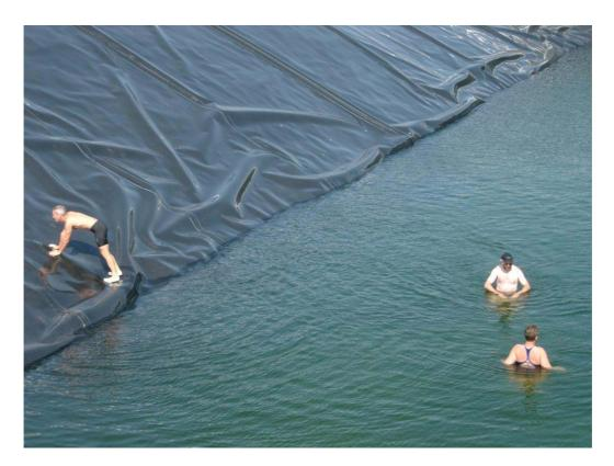
Fig. 2.12. Foldings during filling up.
