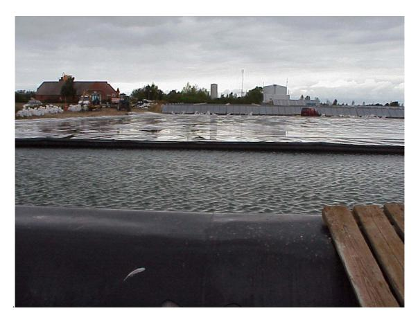
Fig. 2.14. The top-liner nearly drawn over the water.
